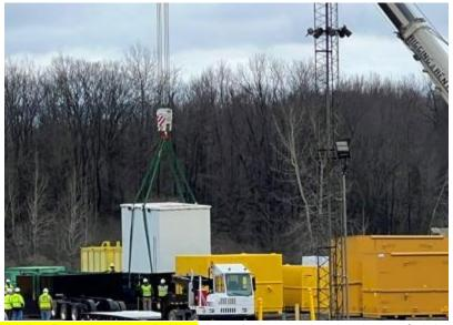
Workers at the West Valley Demonstration Project use a large crane to load one of eight containers of legacy waste into an engineered overpack for safe shipment to an offsite disposal facility.
