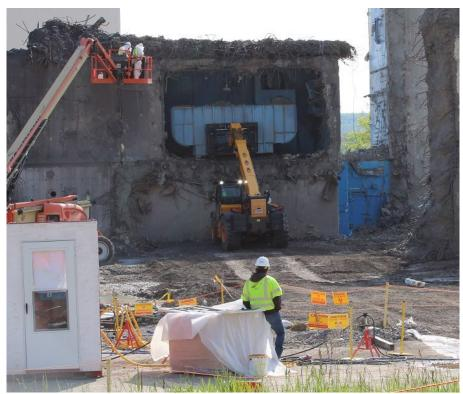
An operator uses a fork truck to safely remove a vent washer from the west side of the Main Plant Process Building at the West Valley Demonstration Project.
