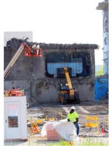
An operator uses a fork truck to safely remove a vent washer from the west side of the Main Plant Process Building at the West Valley Demonstration Project.
