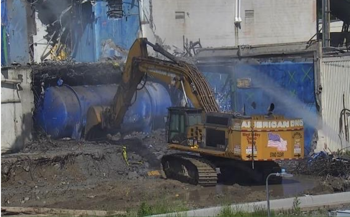
Removal of the Uranium Product Cell Tank 5D-15B from the east side of Main Plant
