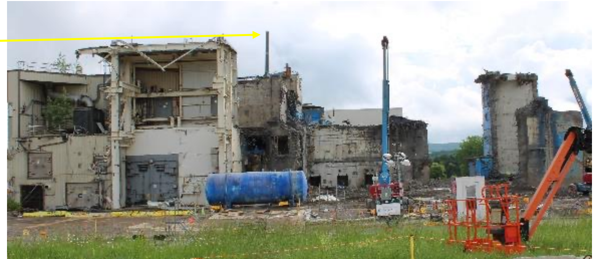
Main Plant west wall (May 2024)
