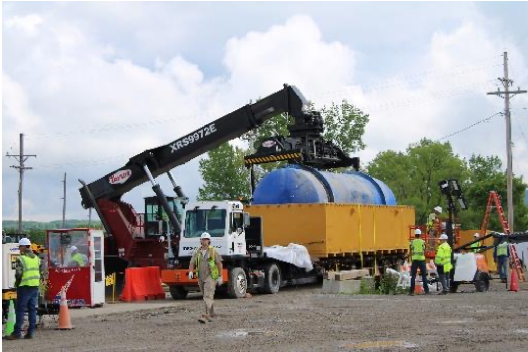
Loading Tank 5D-15B into a specialty container
