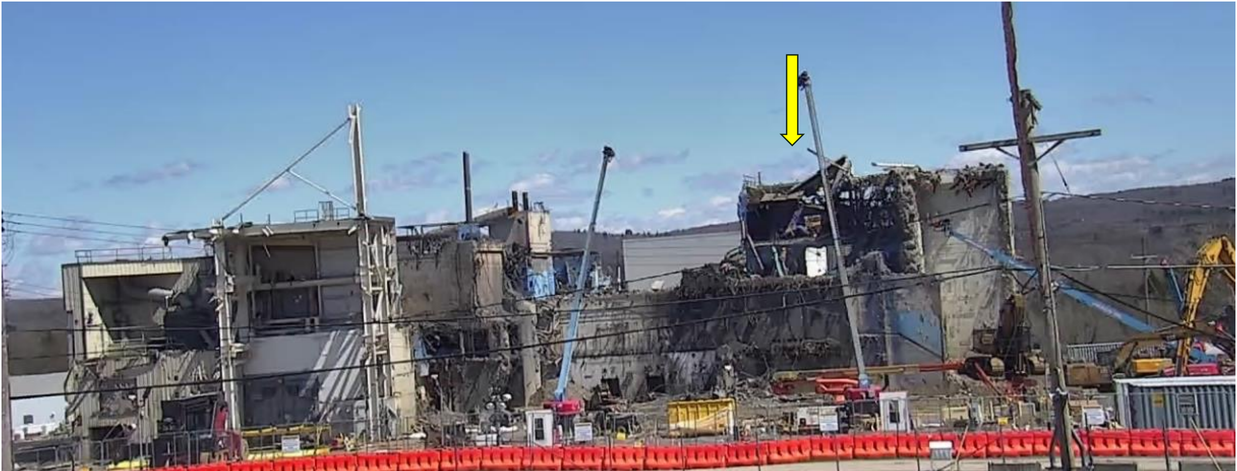
Deconstruction of Control Room and Upper Extraction Aisle
