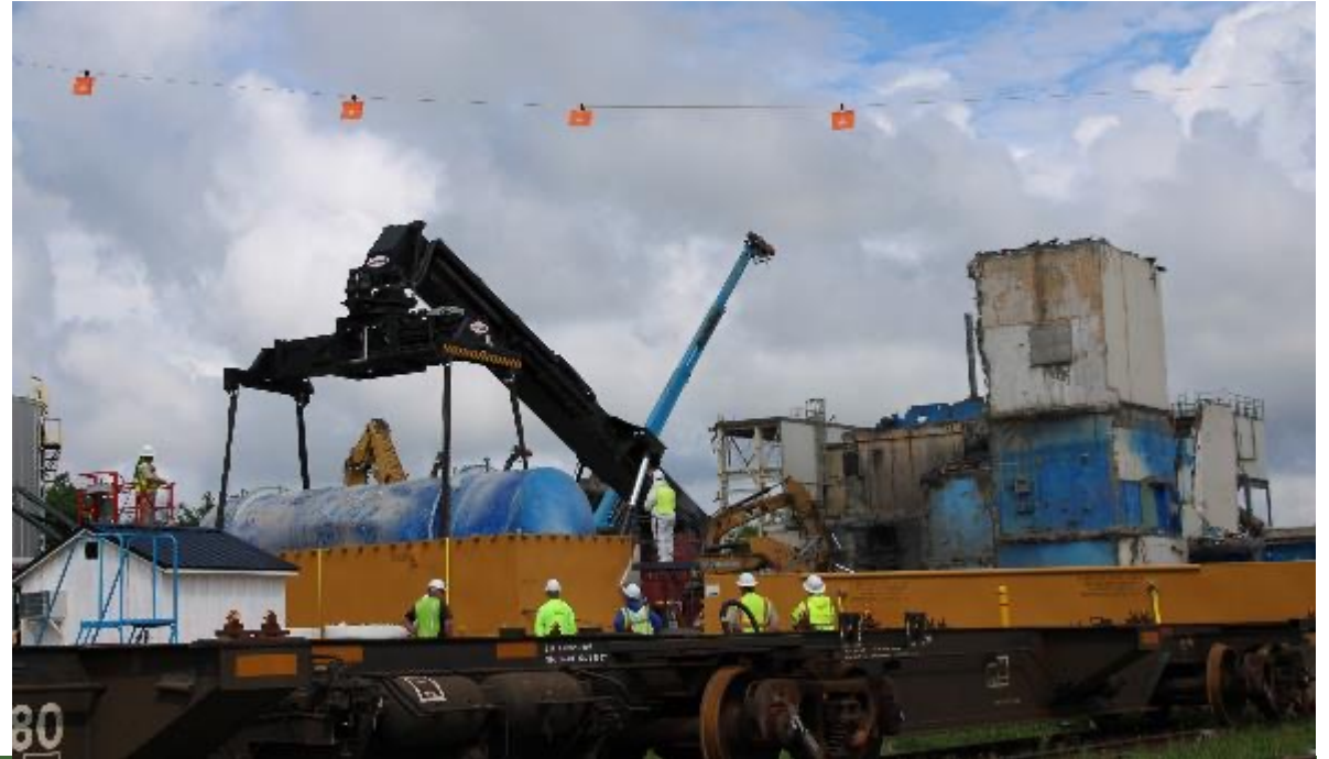
Loading Tank 5D-15B into a specialty container
