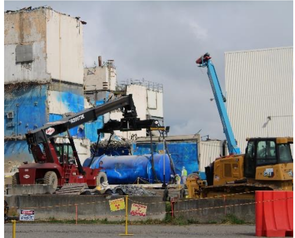
Rigging Tank 5D-15B for placement into specialty shipping container
