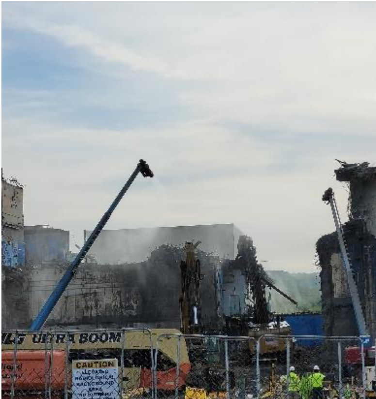
Removal of Liquid Waste Cell and Lower Extraction Aisle (West side)
