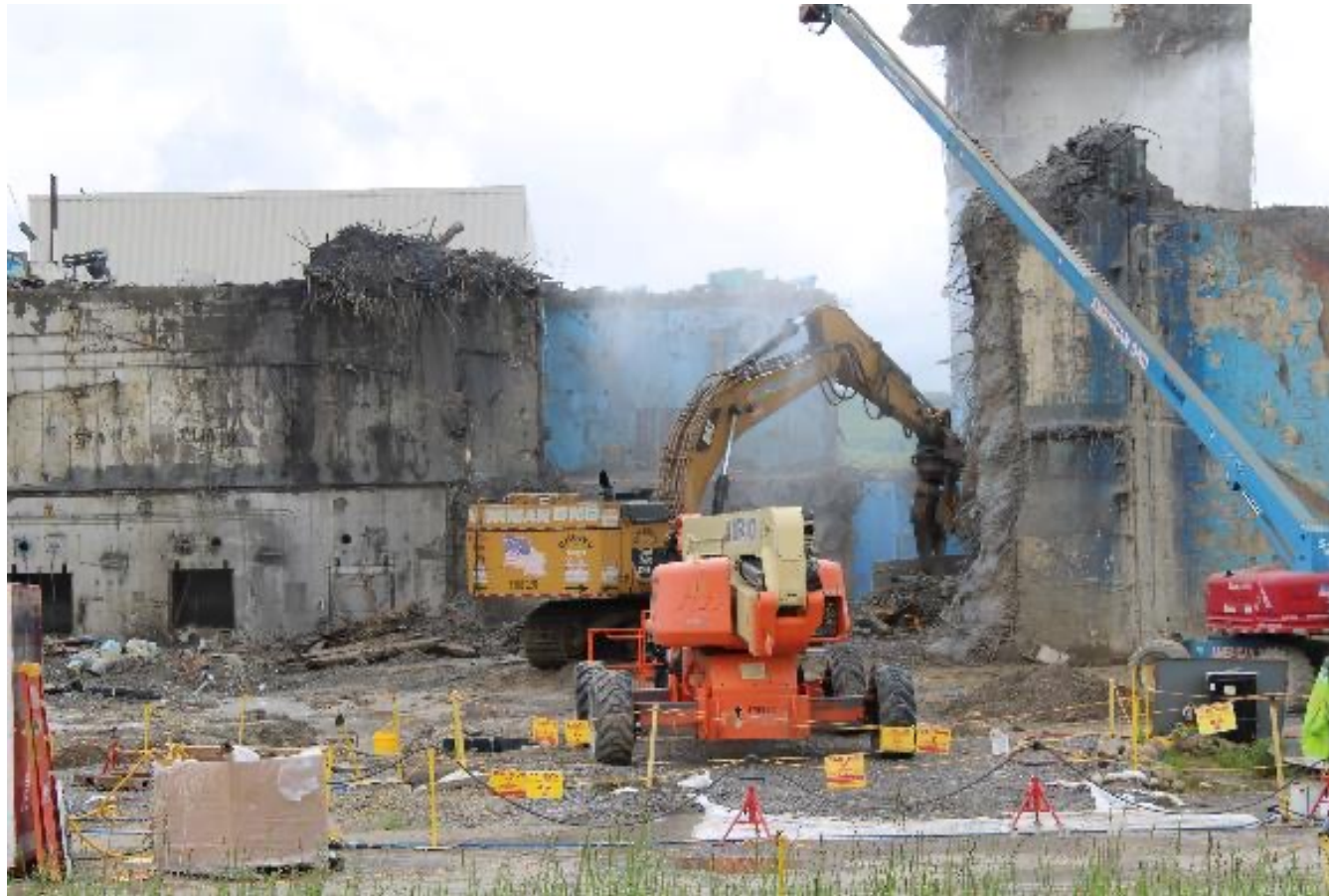
Waste loadout on west side
