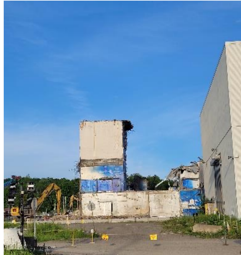
See through building from east side to west side
