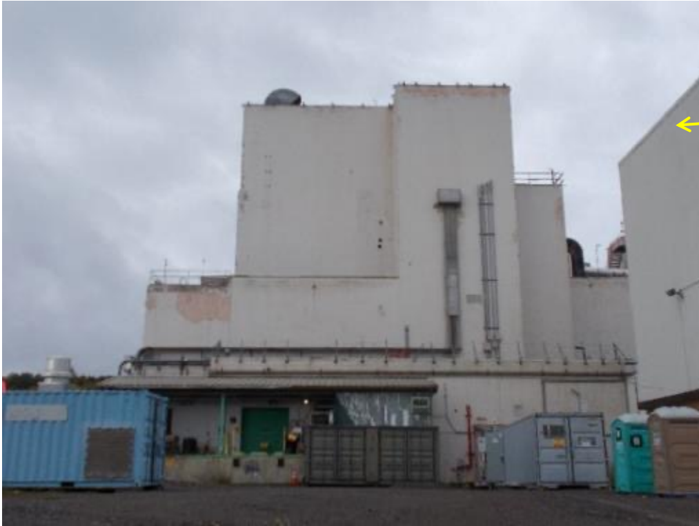
Main Plant east side before deconstruction
