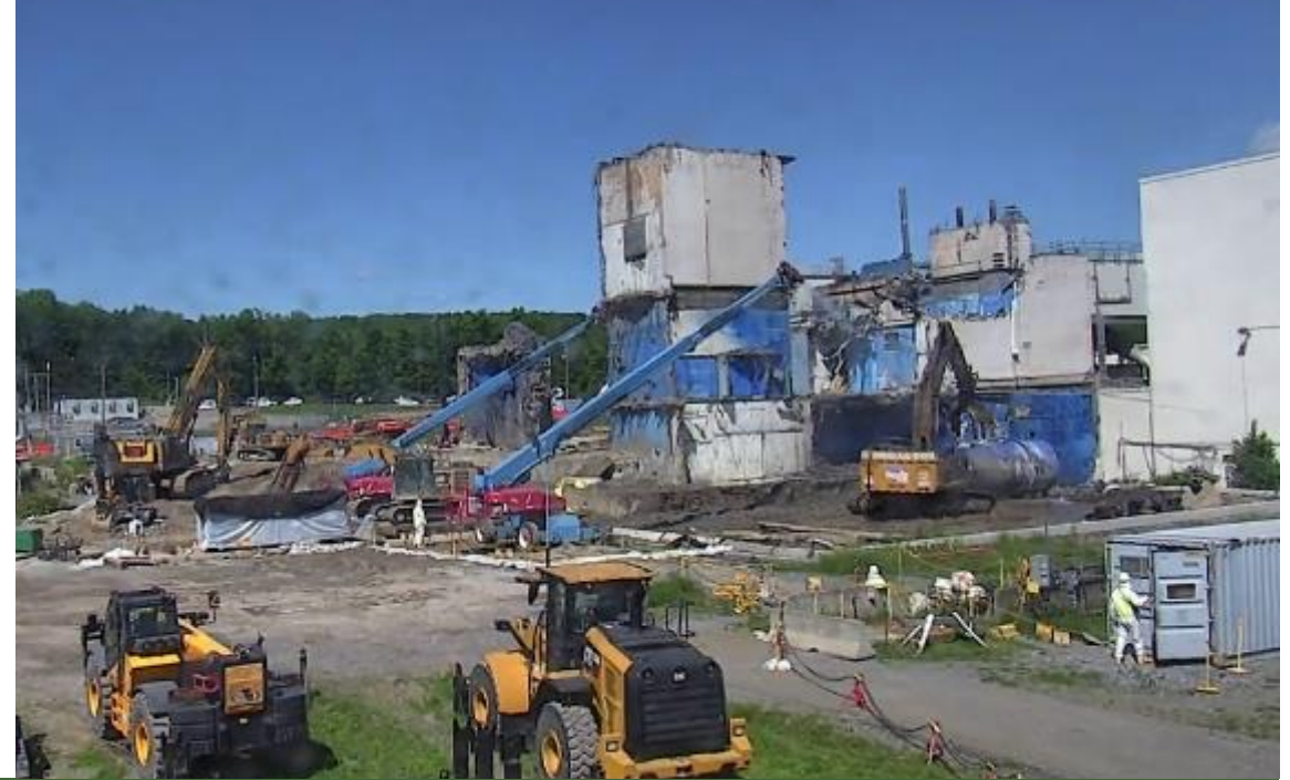
Removal of the Uranium Product Cell Tank 5D-15B from the east side of Main Plant
