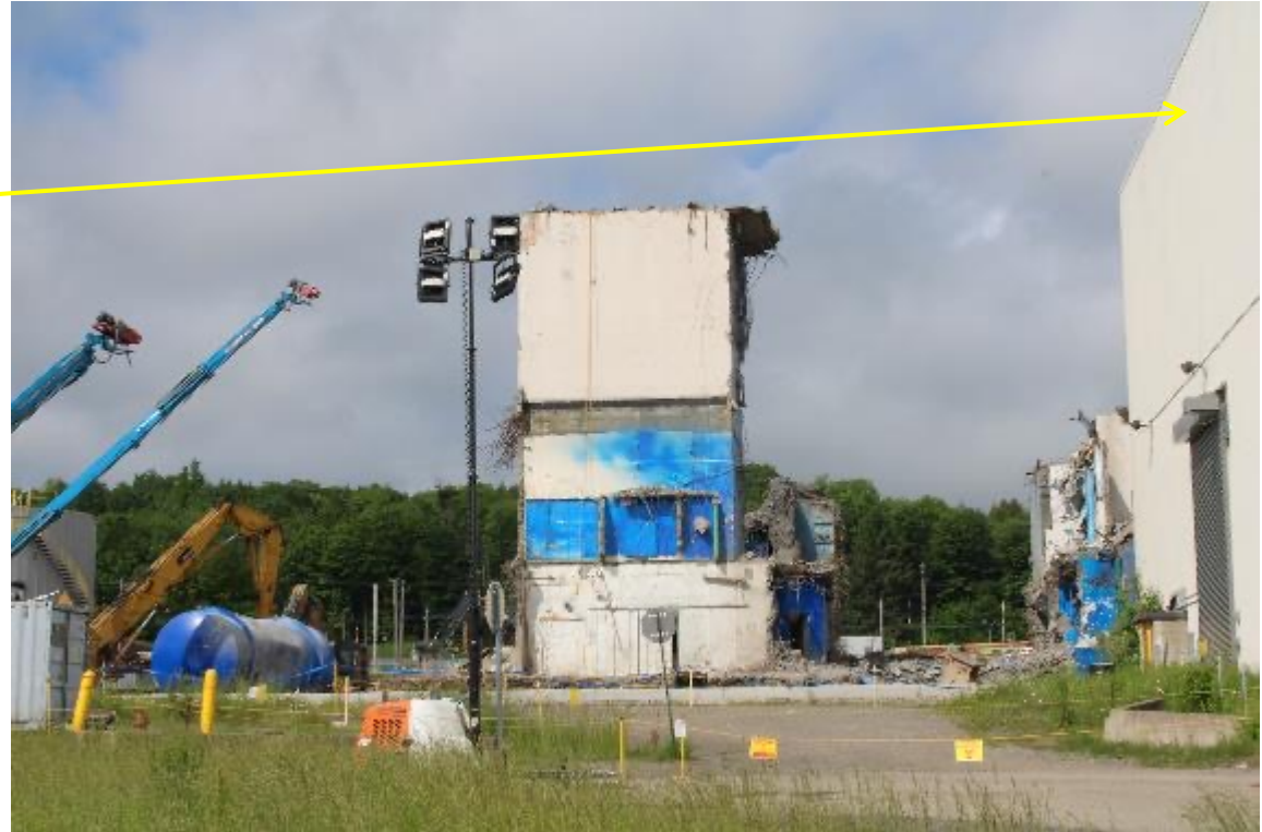
Main Plant east wall (May 2024)
