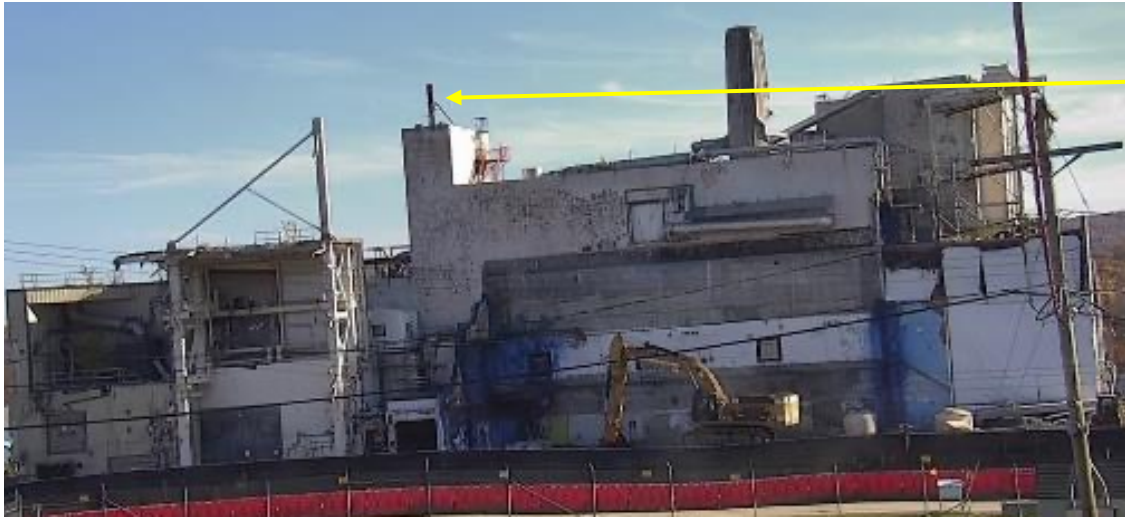
Main Plant west wall before deconstruction (June 2022)
