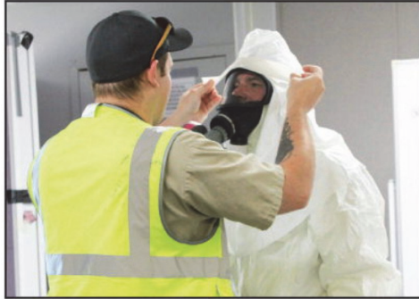
West Valley Demonstration Project Alex Steiner helps Steve Martin suit up in layers of protective clothing before entering the Main Plant Process Building work area.
