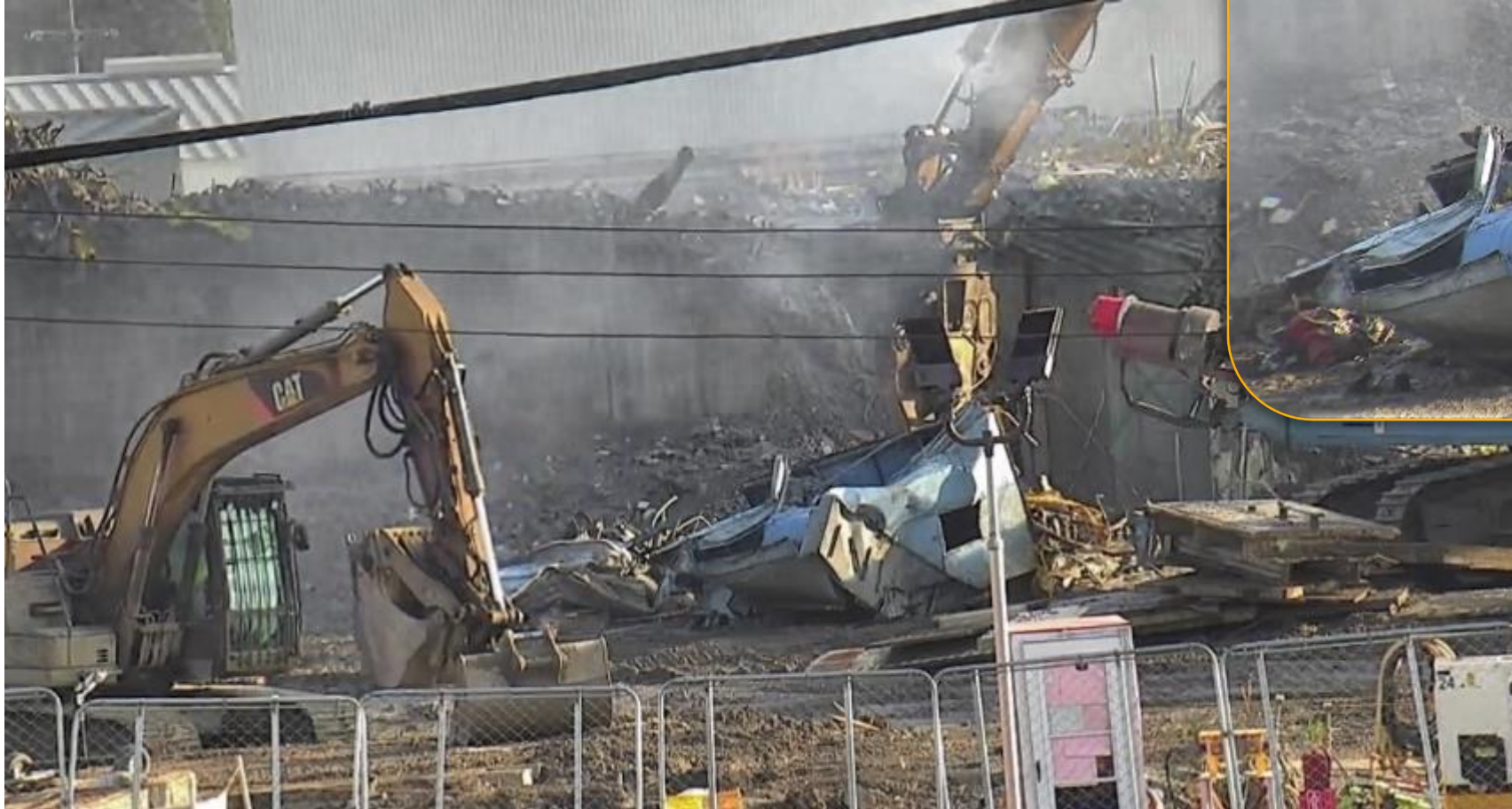
Removal of the Vent Supply Room Supplied Air Plenum
