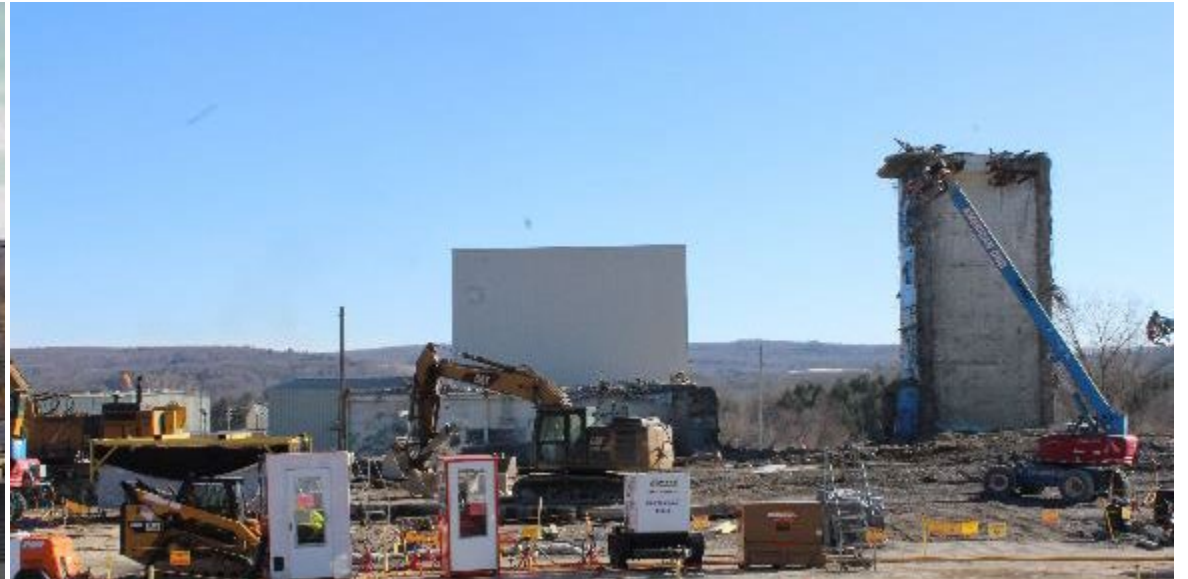
Main Plant west wall (March 2025)
