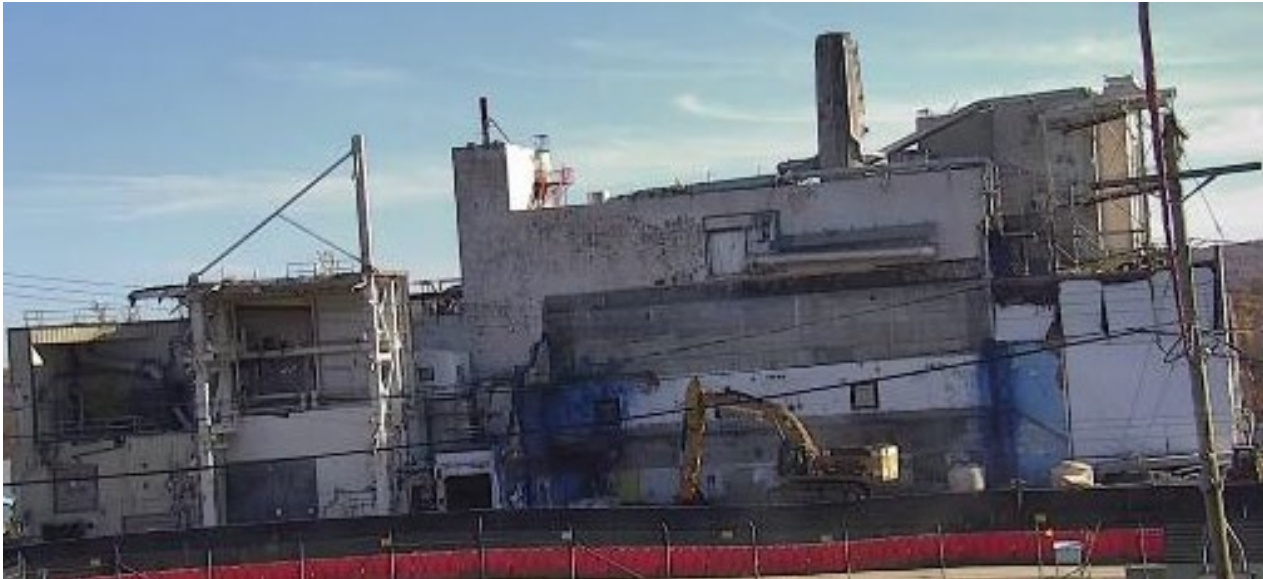
Main Plant west wall before deconstruction (June 2022)
