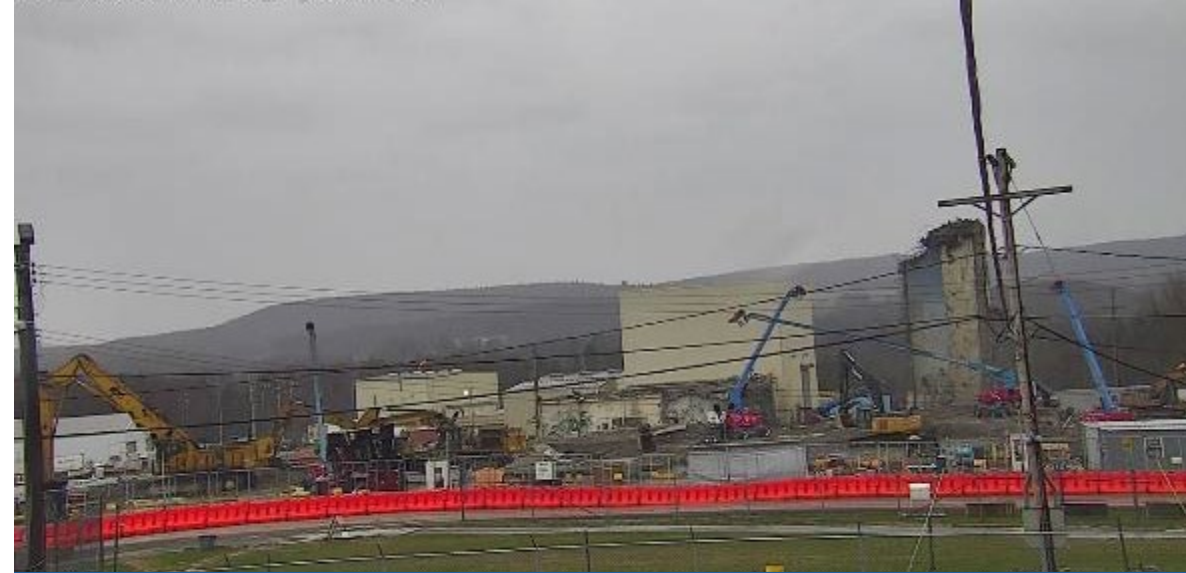
Main Plant west side after deconstruction (April 2025)
