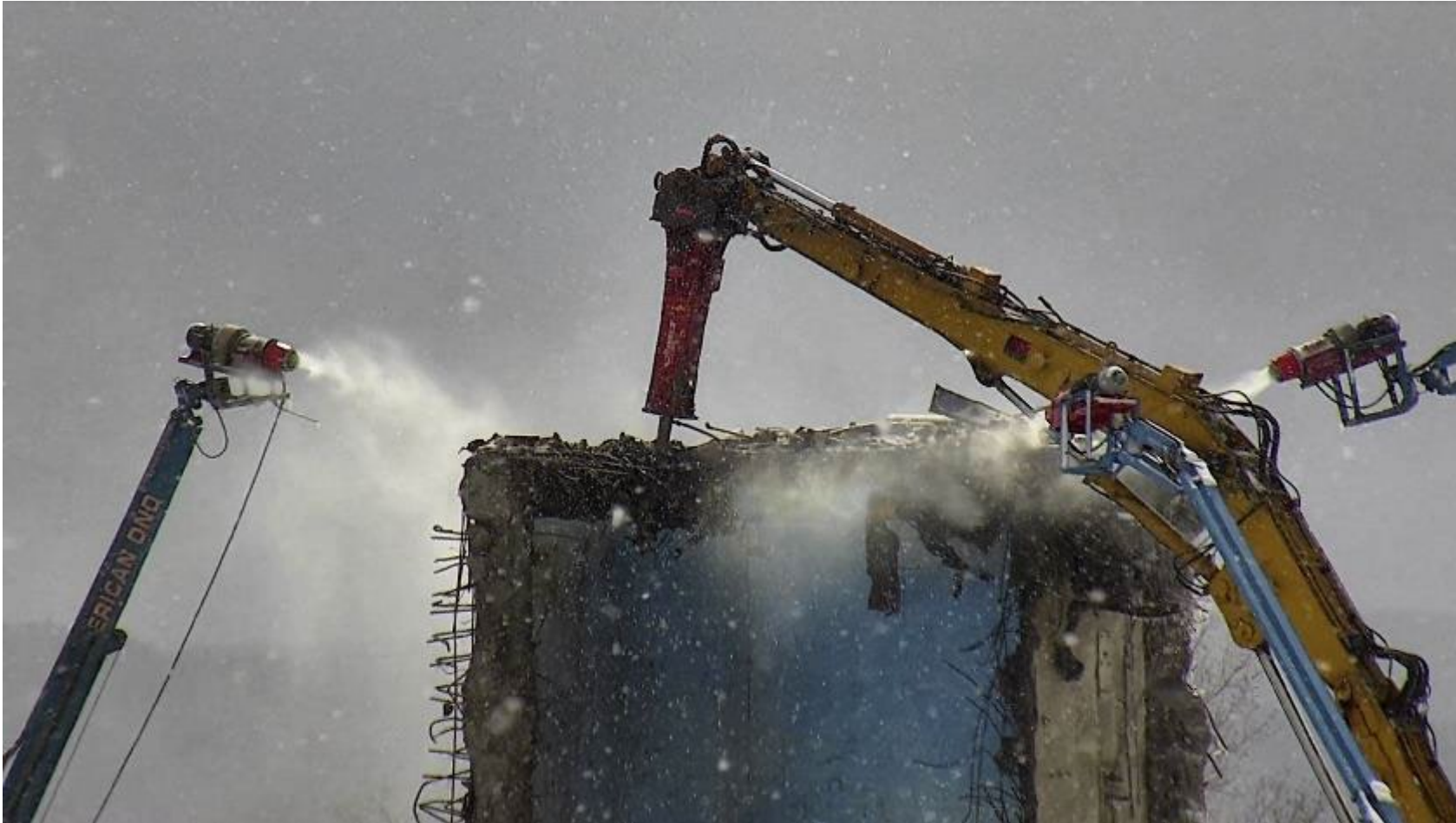
Deconstructing PPC with a hydraulic hammer, and turbomisters for dust suppression
