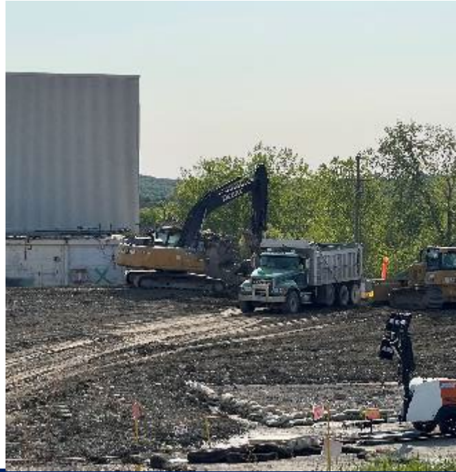
Groundwork for installing the cover (moisture barrier) over the Main Plant Process Building footprint
