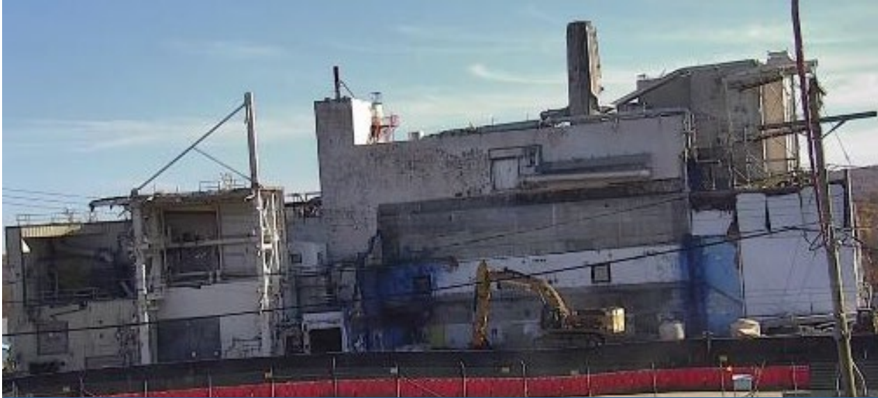
Main Plant west side before deconstruction (June 2022)
