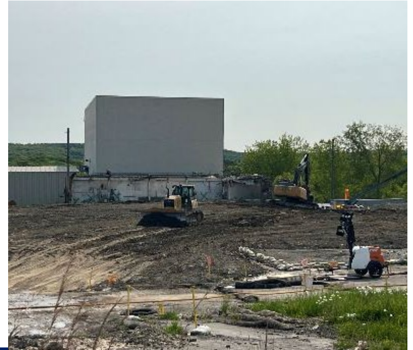
Groundwork for installing the cover (moisture barrier) over the Main Plant Process Building footprint
