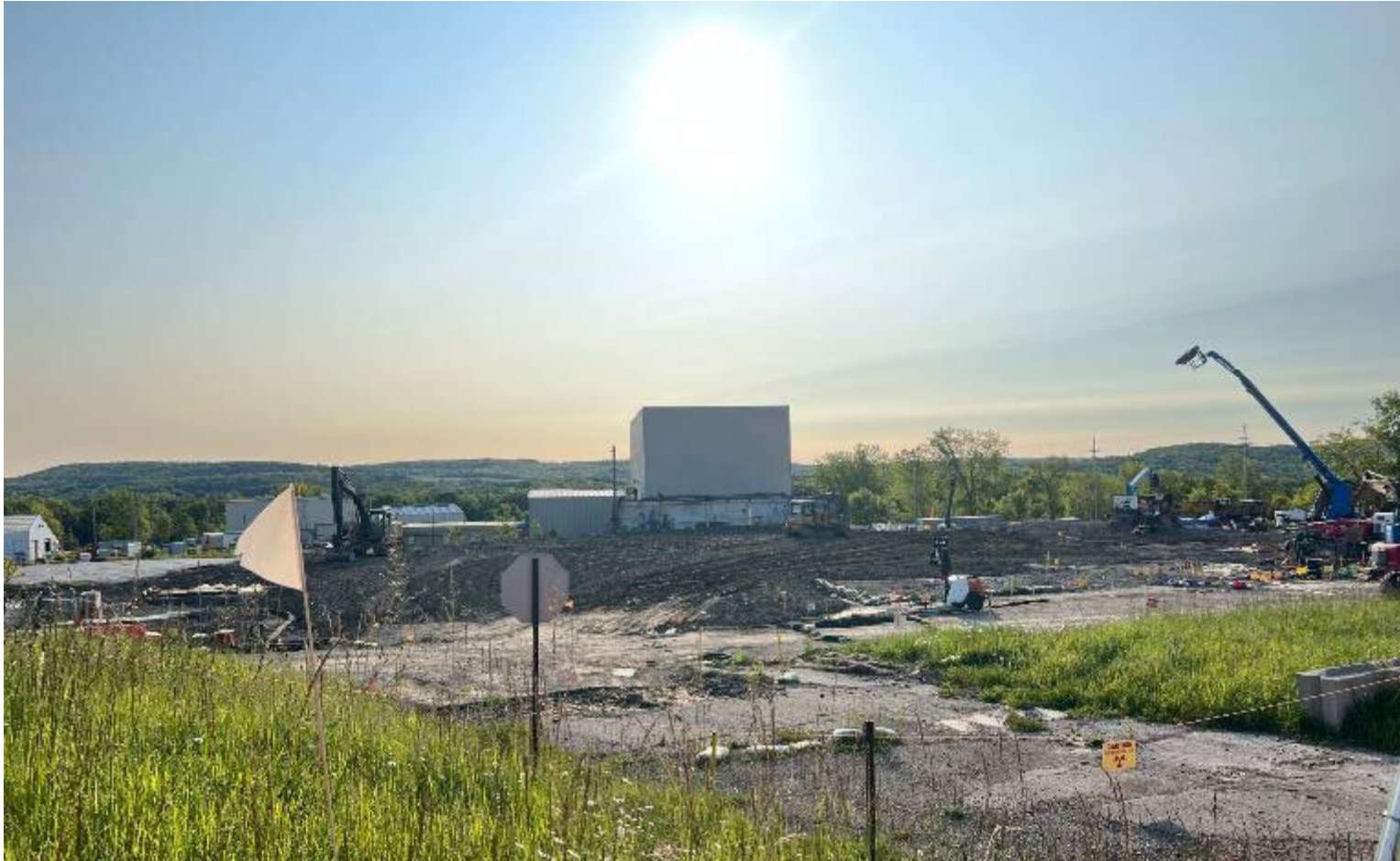
Skyline after the removal of the above-grade portion of Main Plant
