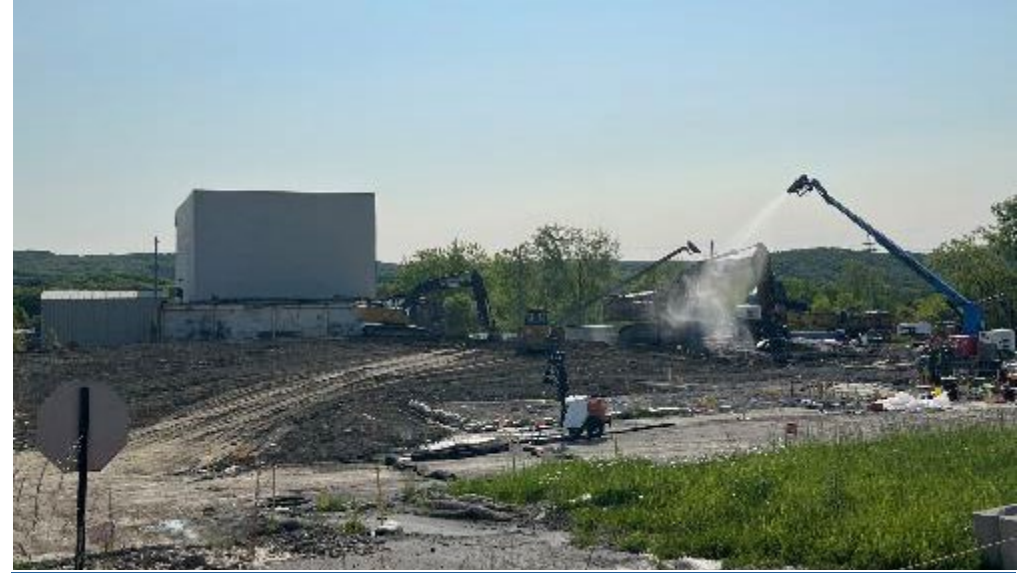
Main Plant west side after deconstruction (June 2025)
