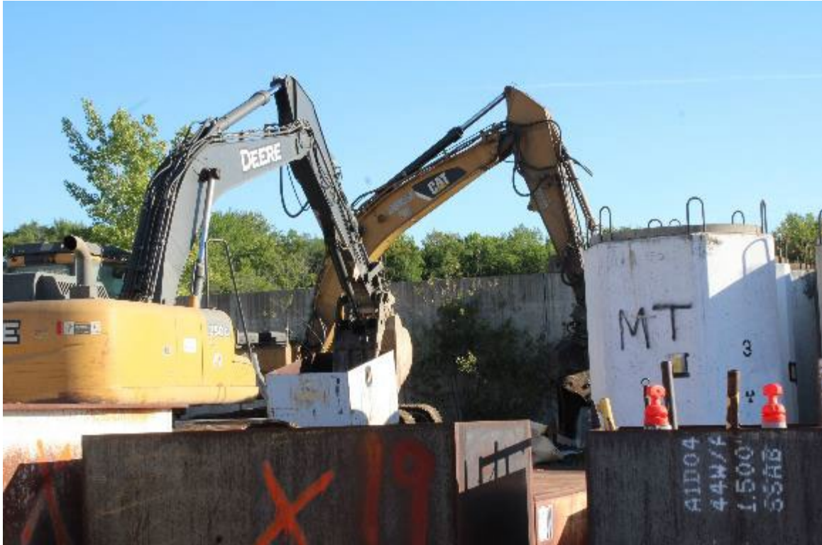
Demolition of legacy liners, containers, and pump storage vaults
