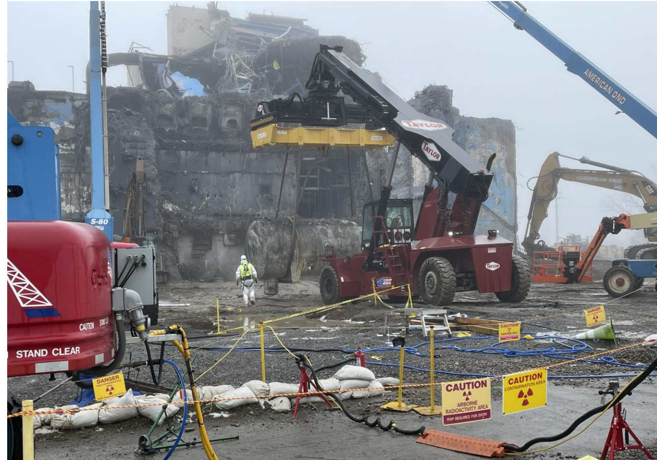
Tank Hoisting and Rigging With Spotters and Cleared Space
