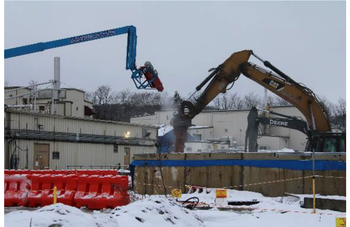
Pump Storage Vault Demolitions – second vault being demolished with hydraulic hammer (front and backside views)
