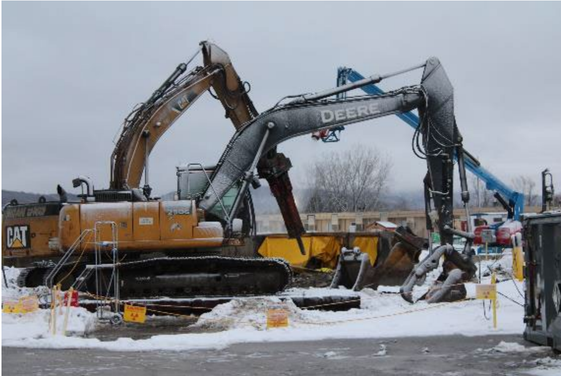
Pump Storage Vault Demolitions – second vault being demolished with hydraulic hammer (front and backside views)
