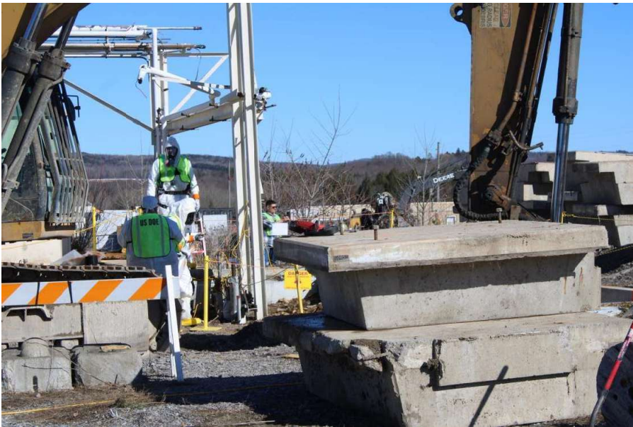
HLW Pipe Trench removal operations
