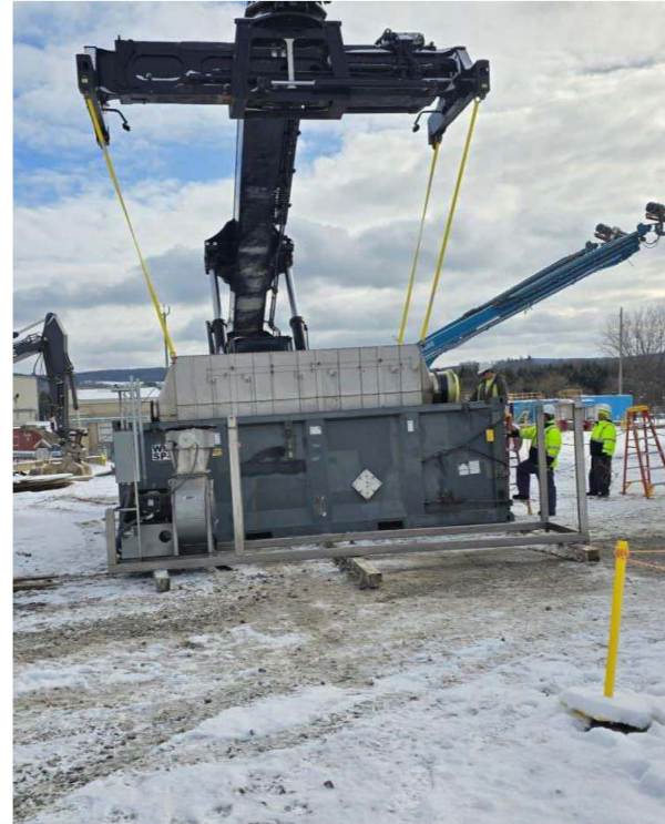
Removal of 1 of 2 Replacement Ventilation Units in preparation for RVU facility demolition
