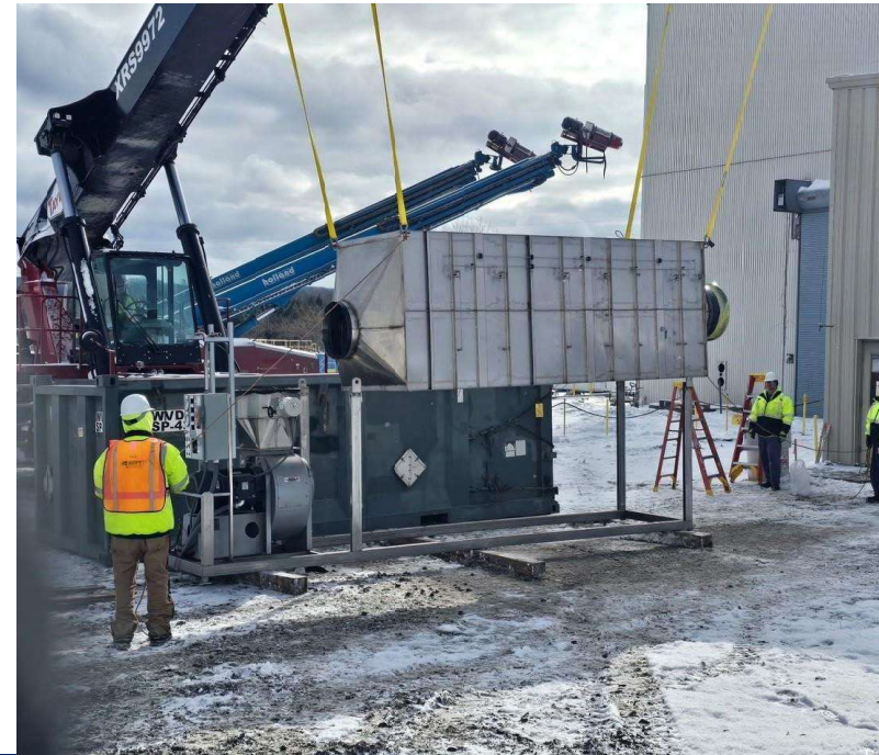
Loading the first RVU into a waste container
