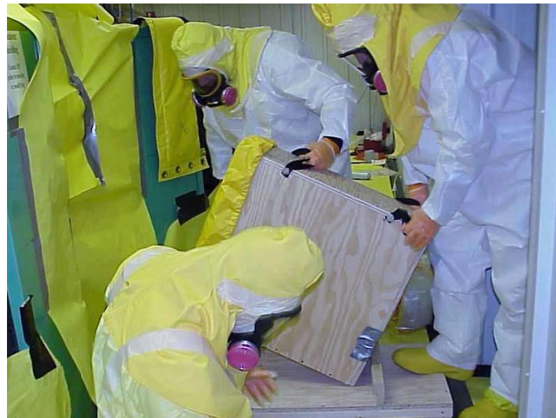
Workers remove lower filter into a box (Cart used for transferring filter box)
