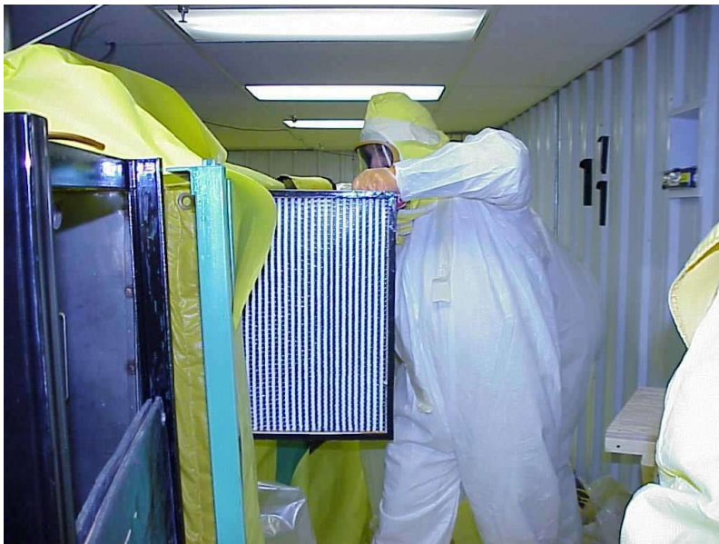
Removal of a South Roughing Filter
