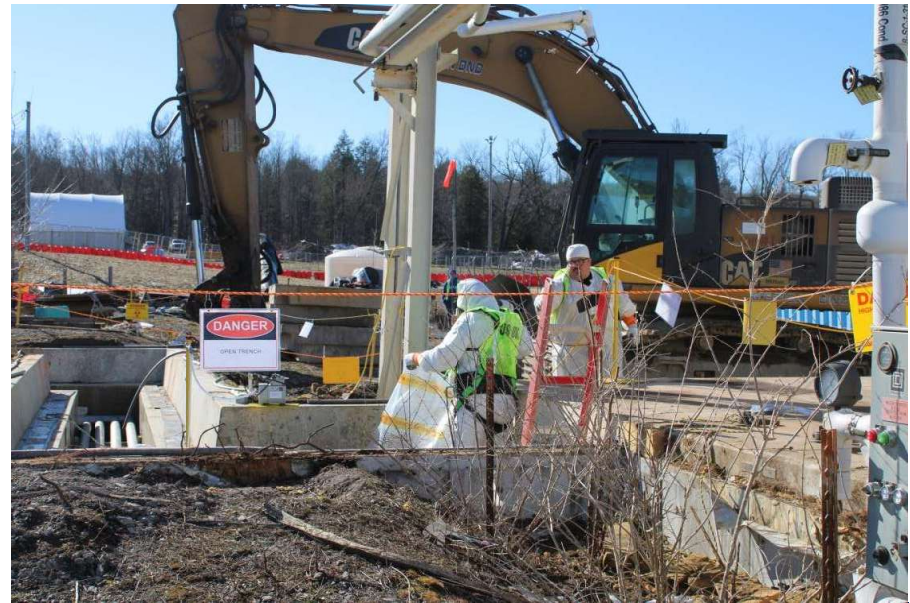
Pipe cutting with support outside work area
