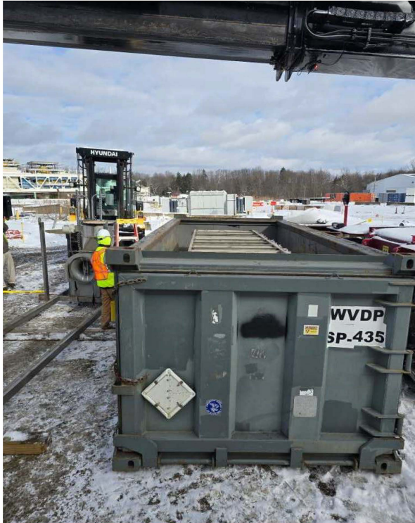
Removal of 1 of 2 Replacement Ventilation Units in preparation for RVU facility demolition
