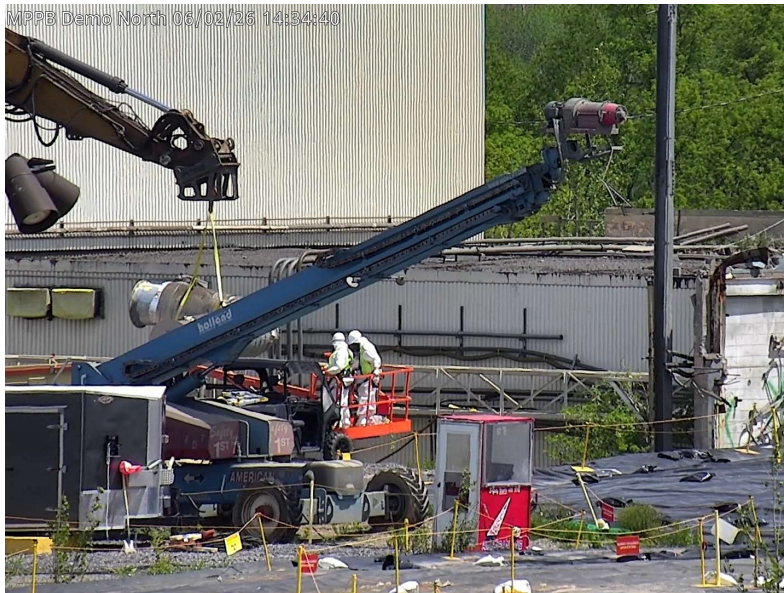
Workers safely remove large ventilation piping from Fuel Receiving & Storage Facility (demolition preparations)
