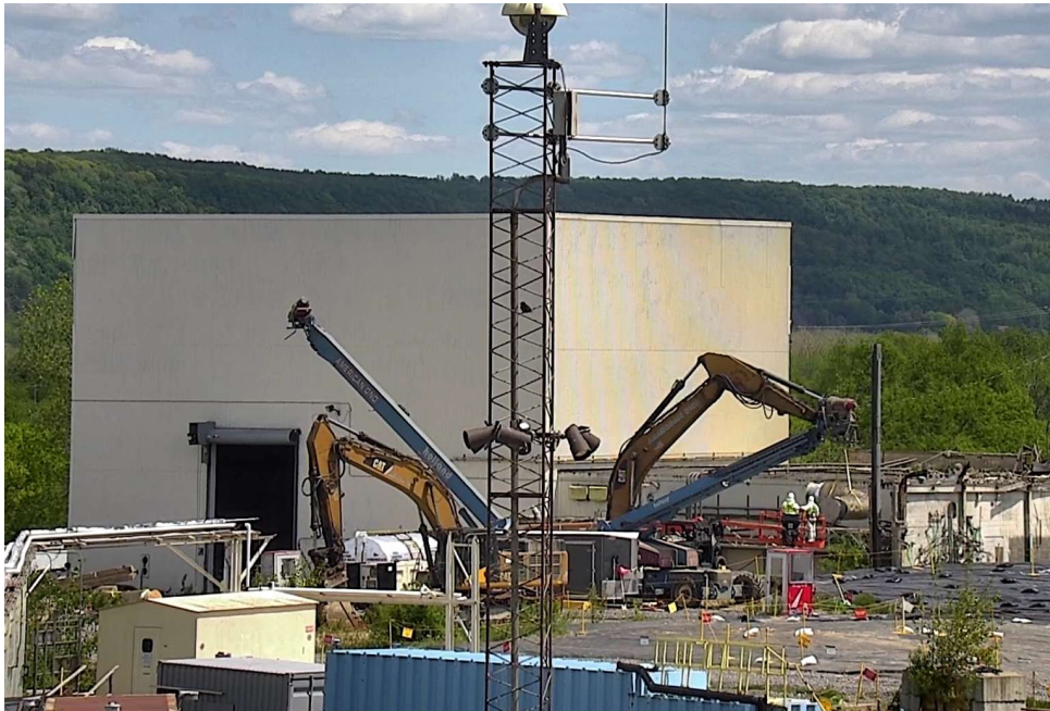
Excavator operator and field workers use teamwork to safely lift large ventilation piping
