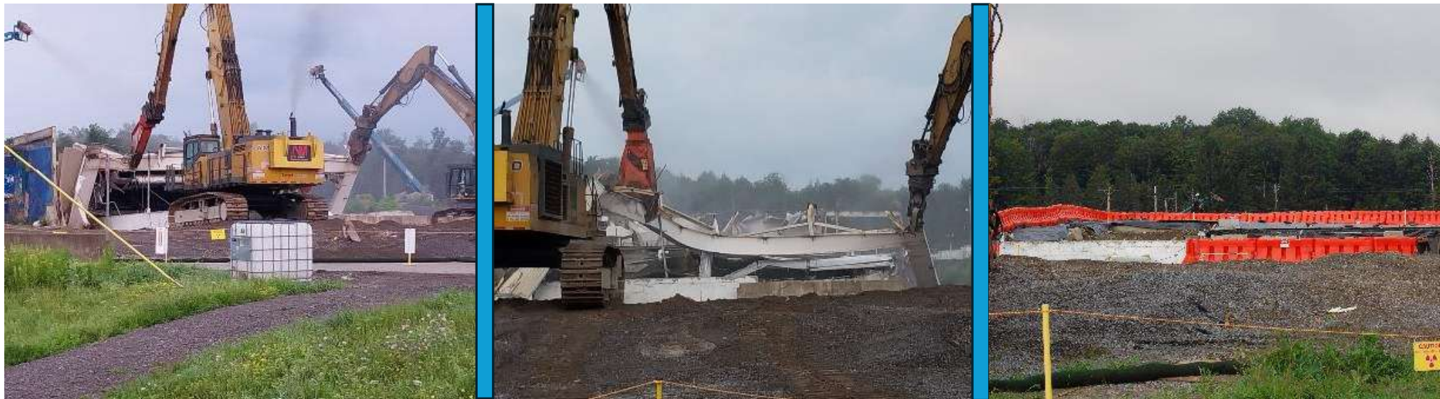
Taking down the FRS lower bay structure to complete demolition
