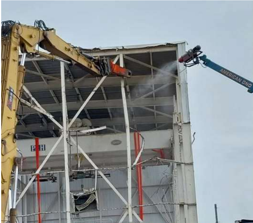
Crews remove the remaining steel beams from the east wall of the FRS
