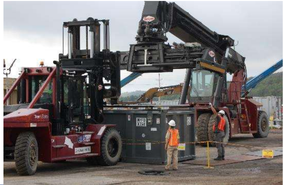
Demolition debris removal: (l) Excavator loads waste container; (r) Heavy-duty fork truck places a lid on the waste container
