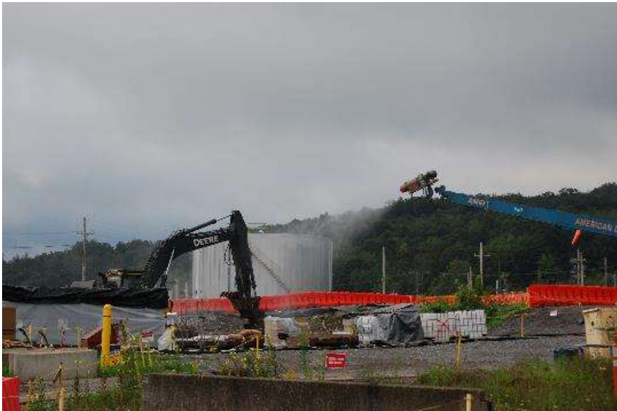
Demolition debris removal: (l) Excavator loads waste container; (r) Heavy-duty fork truck places a lid on the waste container
