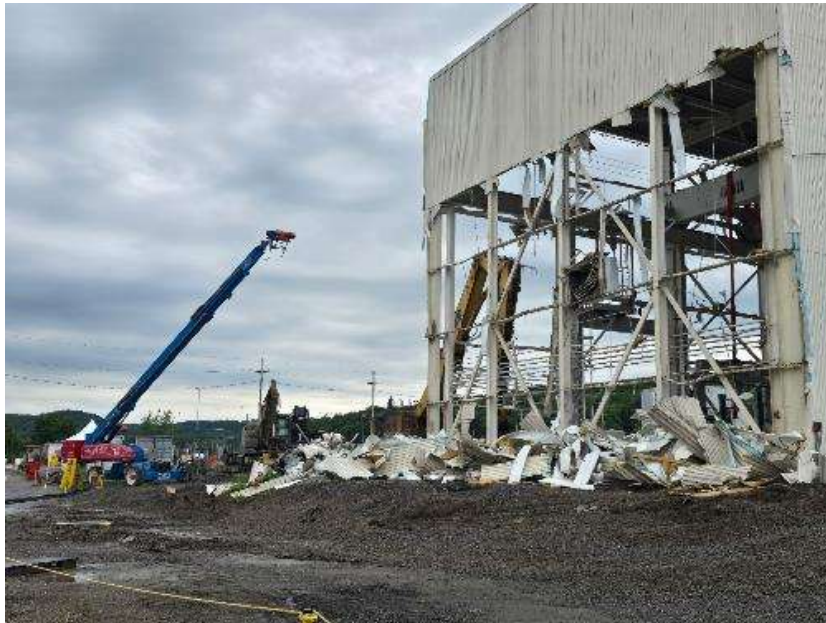
Crews continue to remove the metal exterior of the FRS
