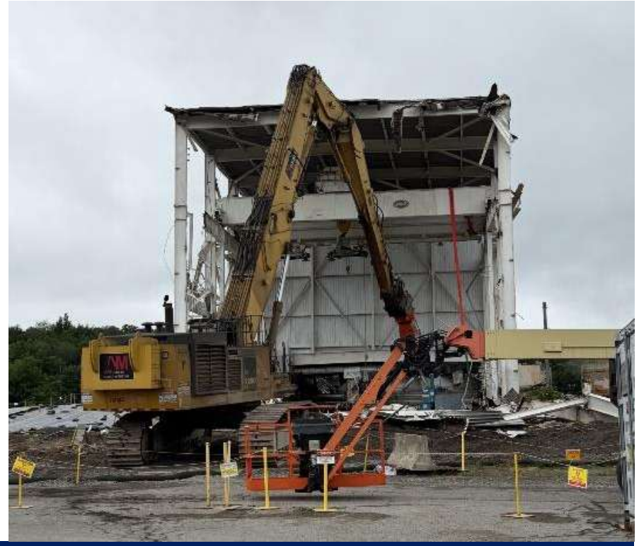
Crews remove the remaining steel beams from the east wall of the FRS
