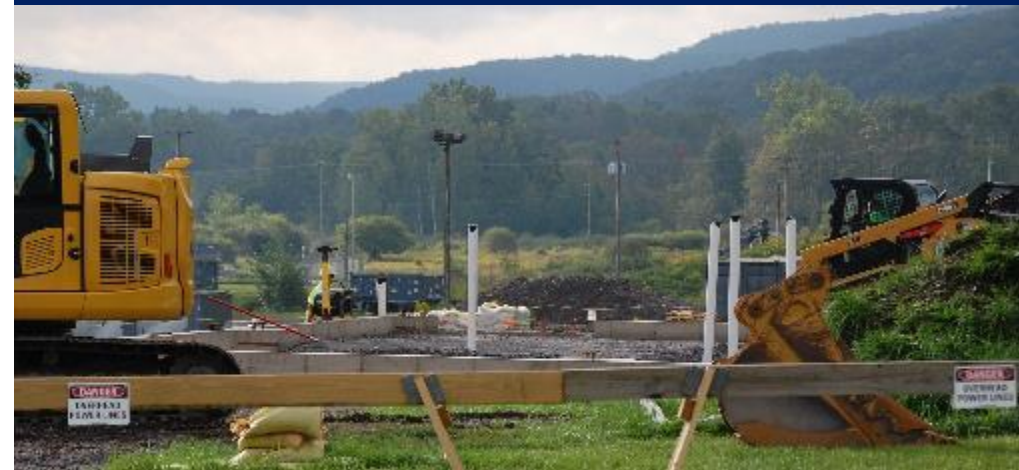
Started the excavation for the Fire Pump House footer
