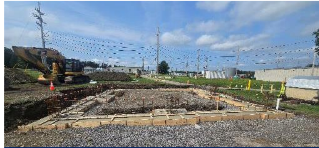
Started the excavation for the Fire Pump House footer
