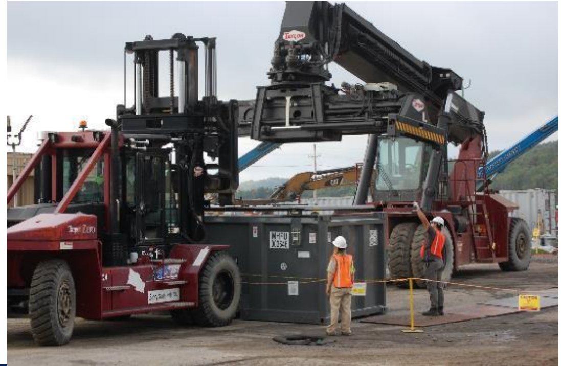
Demolition debris removal: (l) Excavator loads waste container; (r) Heavy-duty fork truck places a lid on the waste container
