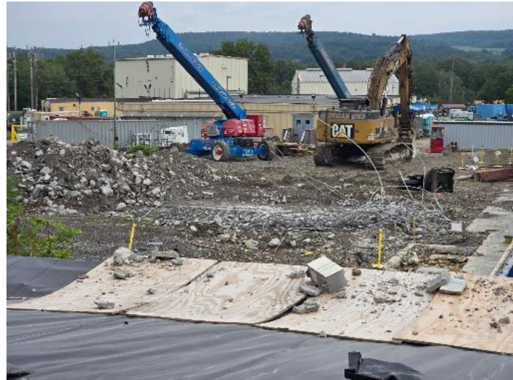
RVU slab demolition (this work will help pave the way for Waste Management Area-1 Excavation)
